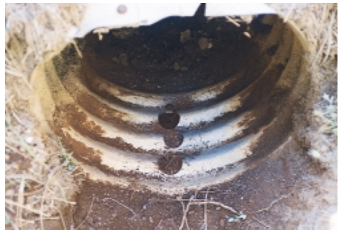
◀ AK Steel Research Center's corrosion engineers and Missouri D.O.T. material engineers inspect a 43-year old Aluminized Steel Type 2 pipe installation. This is one of two culvert installations in Carter County, Missouri, installed in a series containing half Aluminized Steel Type 2 pipe and half galvanized steel pipe.
