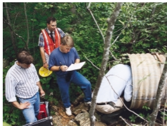
◀ AK Steel Research Center's corrosion engineers and Missouri D.O.T. material engineers inspect a 43-year old Aluminized Steel Type 2 pipe installation. This is one of two culvert installations in Carter County, Missouri, installed in a series containing half Aluminized Steel Type 2 pipe and half galvanized steel pipe.
