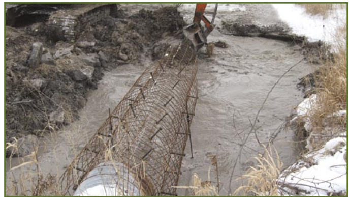
BEAVER STOP® CAN BE ASSEMBLED IN THE SUMMER MONTHS RIGHT AT THE SITE, OR INSIDE A SMALL SHOP DURING THE COLDER MONTHS.
